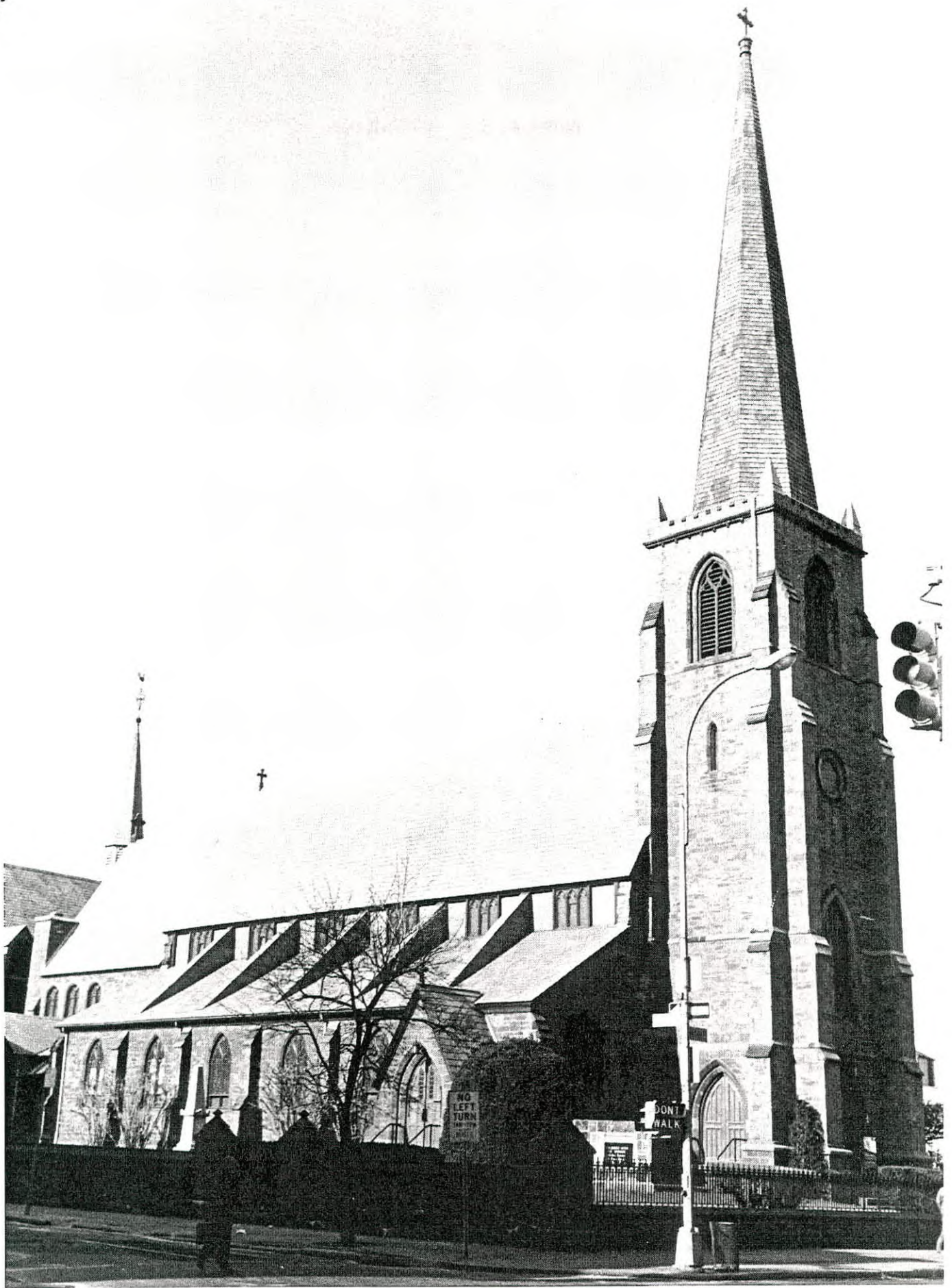
St. George's (Episcopal) Church View from the southeast showing the Main Street and 39 th Avenue facades Photo: LPC, January 1982
