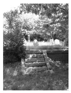
volunteered in and around the wall, further compromising the strength of the wall. It is likely that the original wall was dry laid, and that mortared was added at a later date, trapping water behind the wall
