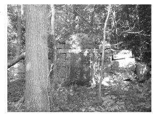
the tomb, contributing the structure's deterioration. One tree has fallen on the tomb to the left of the door. While the door has been sealed with mortared brick, hardware remaining in the door jam area suggests the tomb once had a door.
