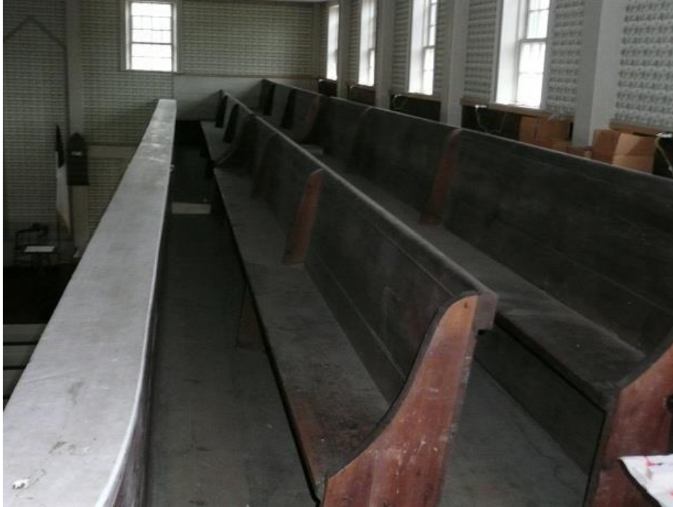
19. Detail of benches in balcony, looking north.
