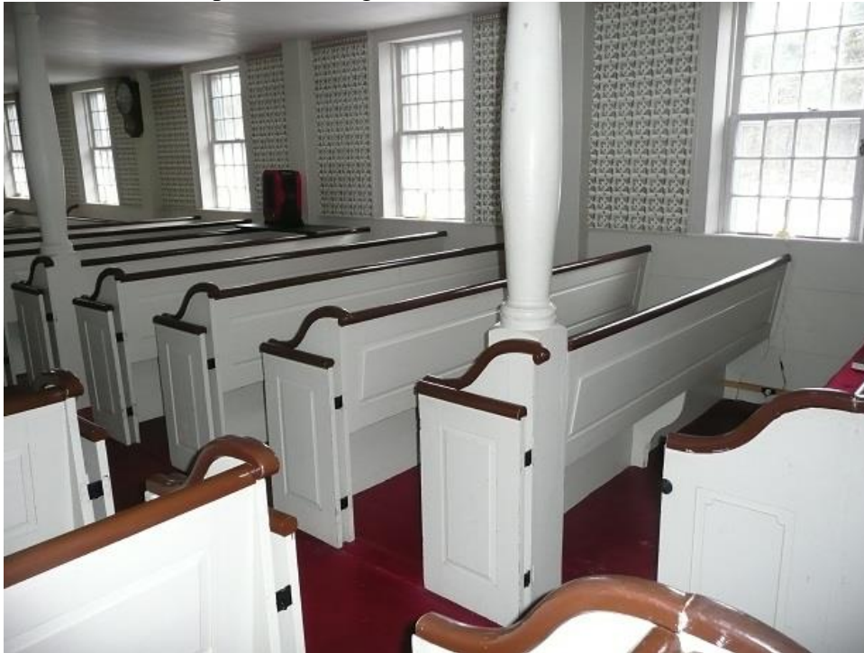
17. Detail of box pews, looking northeast.
