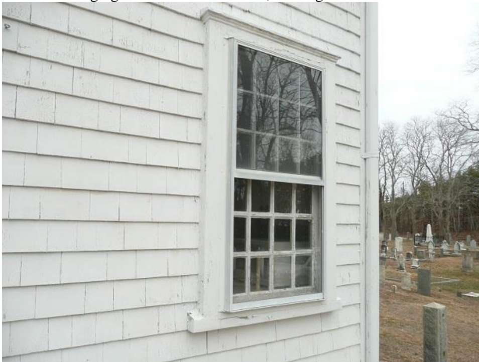
6. First Congregational Parish Window, looking northwest.
