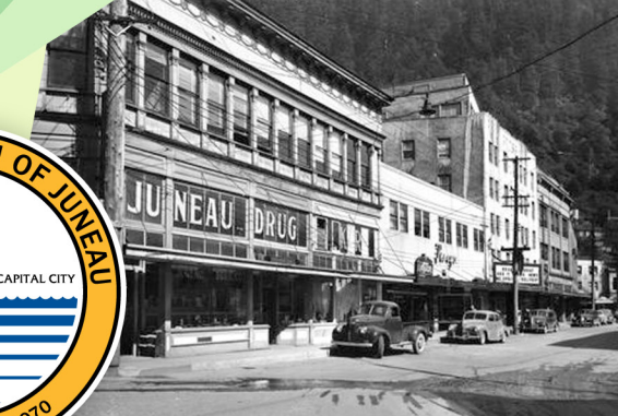
"Valentine Building and the Gross Theater on Front Street ca. 1940" P87-1007 Alaska State Library Winter and Pond Photo Collection
